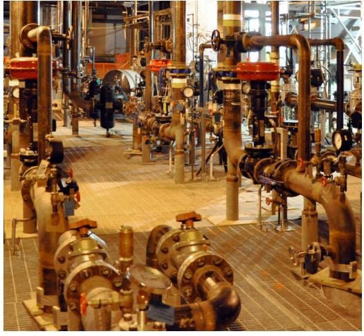
Kurz 534FTB inline flow meters for industrial gas flow measurement are designed to eliminate the need for field fabrication and assembly of inlet and outlet piping sizes by providing accurate gas flow measurement under changing upstream and downstream flow profiles. Built-in reducers/expanders result in exceptional immunity to upstream and downstream flow disturbances caused by valves, bends, and short straight runs.
