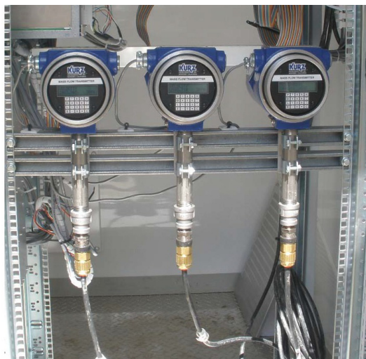
Figure 2-21. Cable gland example with braided shielded cable
